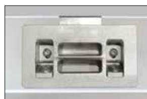
Ventilation position. The striking plate allows a 5mm night ventilation opening for all espagnolette handles.
